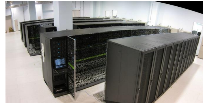
December 2011 - Ready to run acceptance complete
