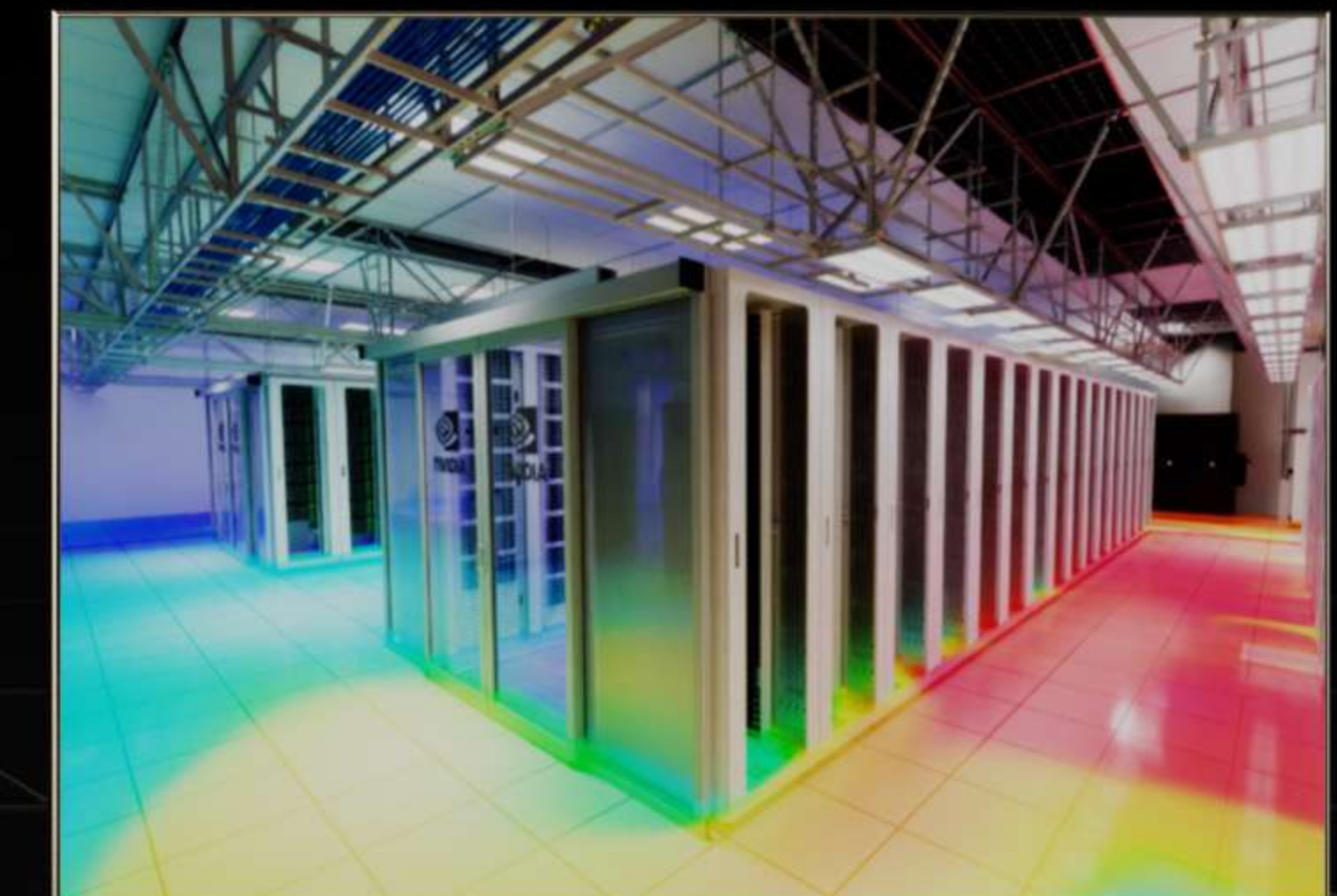
INDUSTRIAL DIGITAL TWIN Data Center CFD Acceleration
